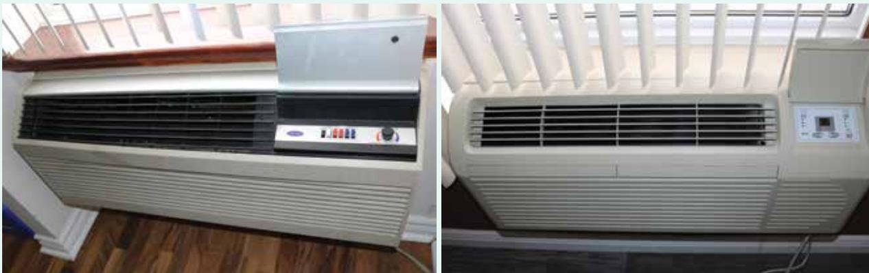
Old air-conditioning unit (left) at the Peninsula Inn Hotel in Niagara Falls switched for an energy efficient packaged terminal heat pump unit (right) under the pilot.
