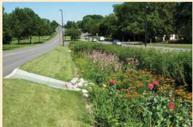
Example of a bioswale to increase water absorption in a highway median.
