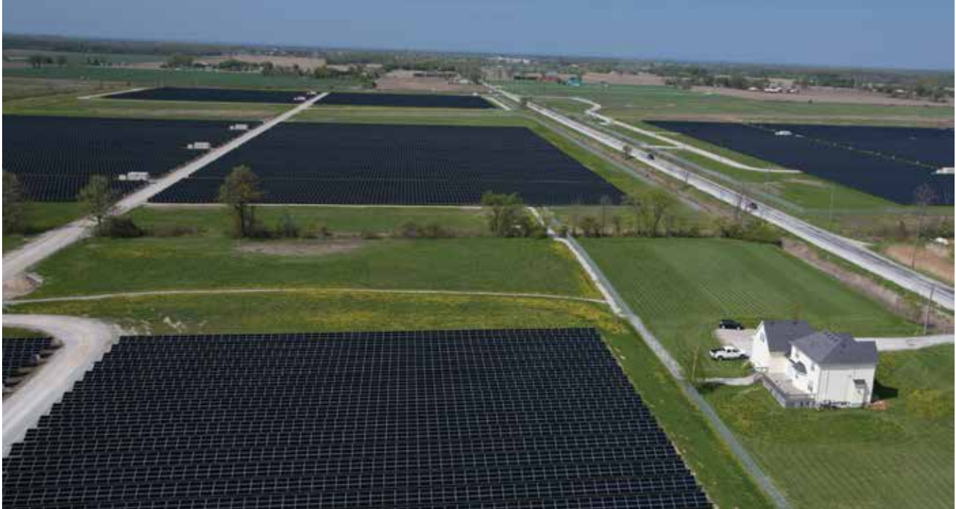
Solar farms generate clean electricity but occupy a large land area (Enbridge solar farm in Sarnia).
