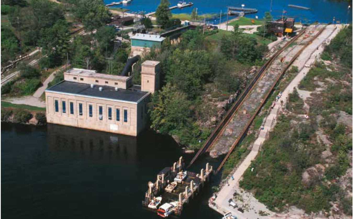
Multiple use of waterways for hydropower and navigation – Big Chute on the Trent-Severn Waterway.
