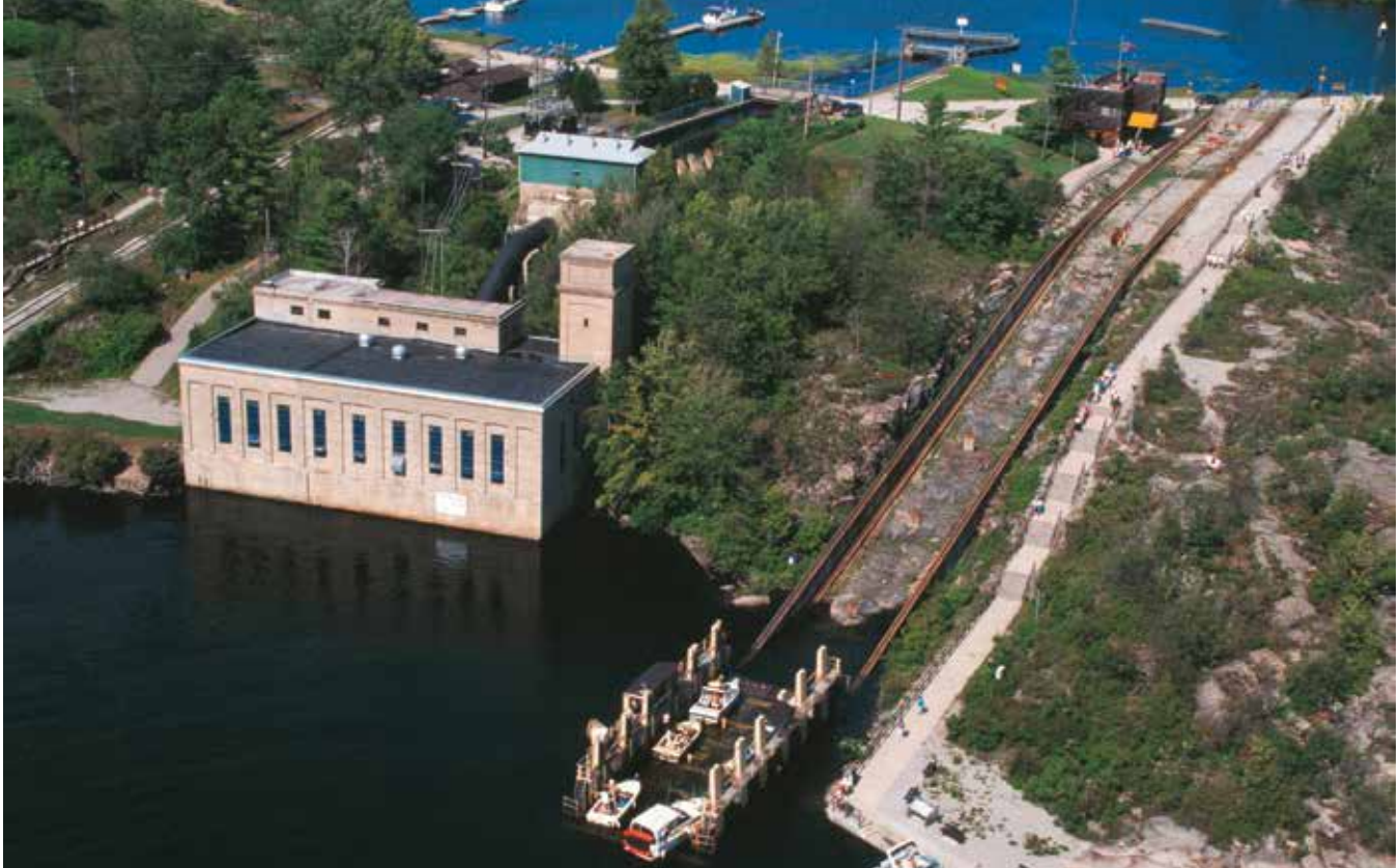
Multiple use of waterways for hydropower and navigation – Big Chute on the Trent-Severn Waterway.
