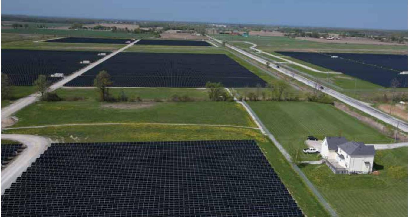
Solar farms generate clean electricity but occupy a large land area (Enbridge solar farm in Sarnia).
